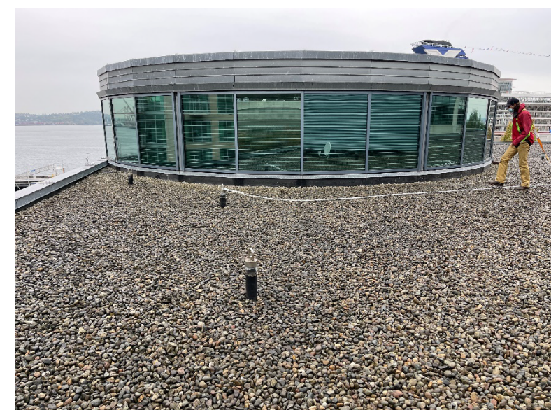
WTCW Roof Photos of Existing Gravel Ballast and Membrane
